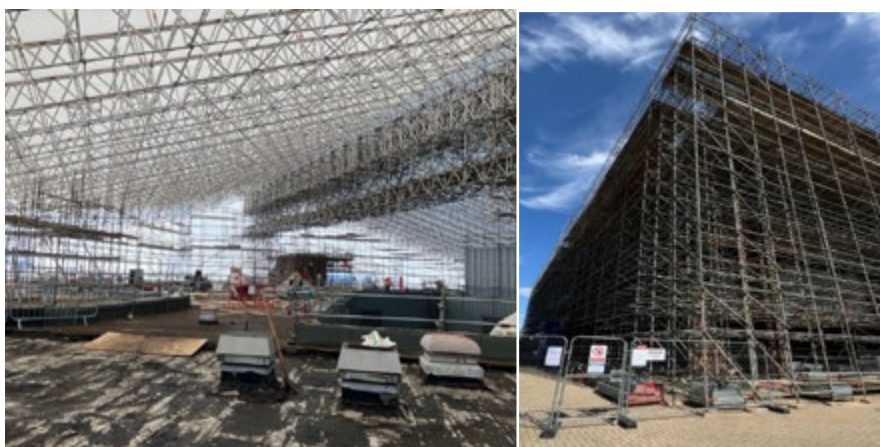
Scaffolding at Harrow Crown Court.
