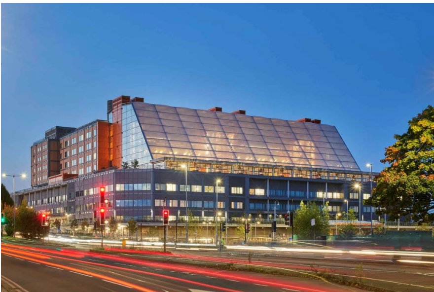
Figure 3: Midland Metropolitan University Hospital, opened October 2024
