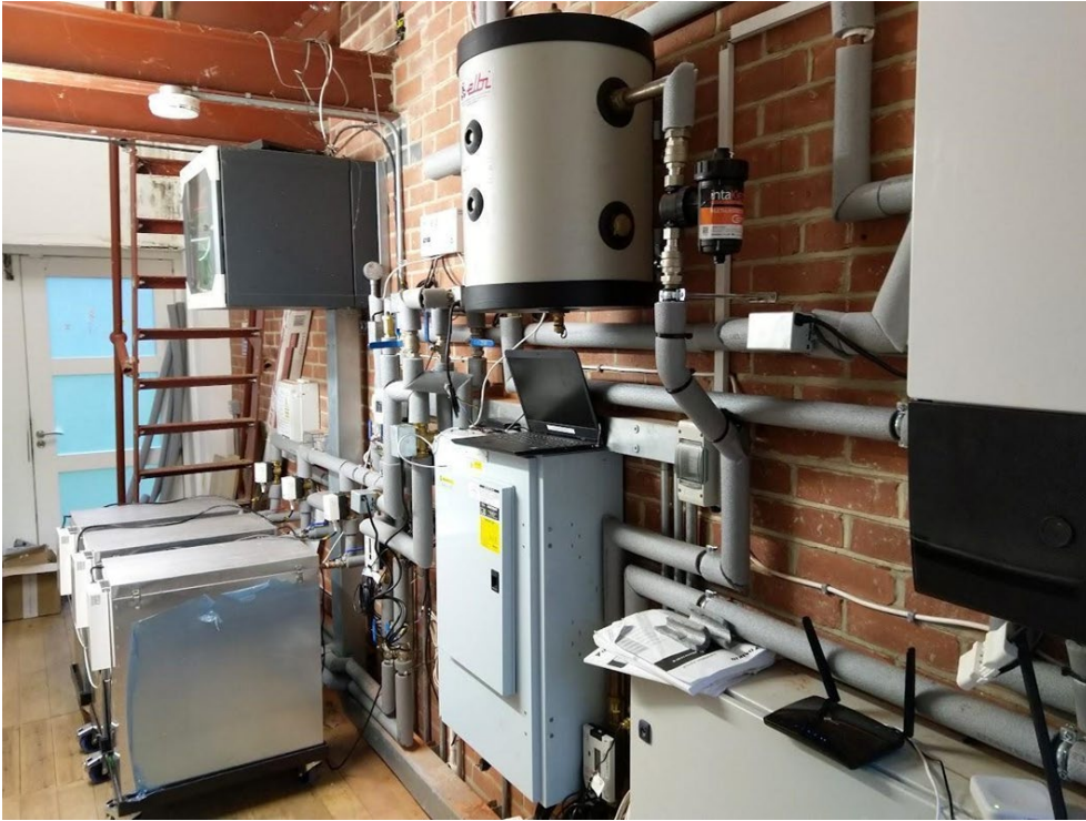
Figure 12: PCM thermal stores installed into the 1930s house.
