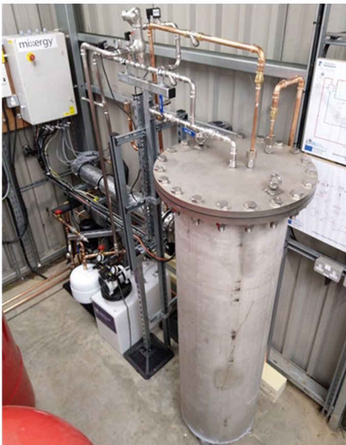
Figure 51: Completed installation of the Gen 1 store into the DHN shed, prior to insulation.
