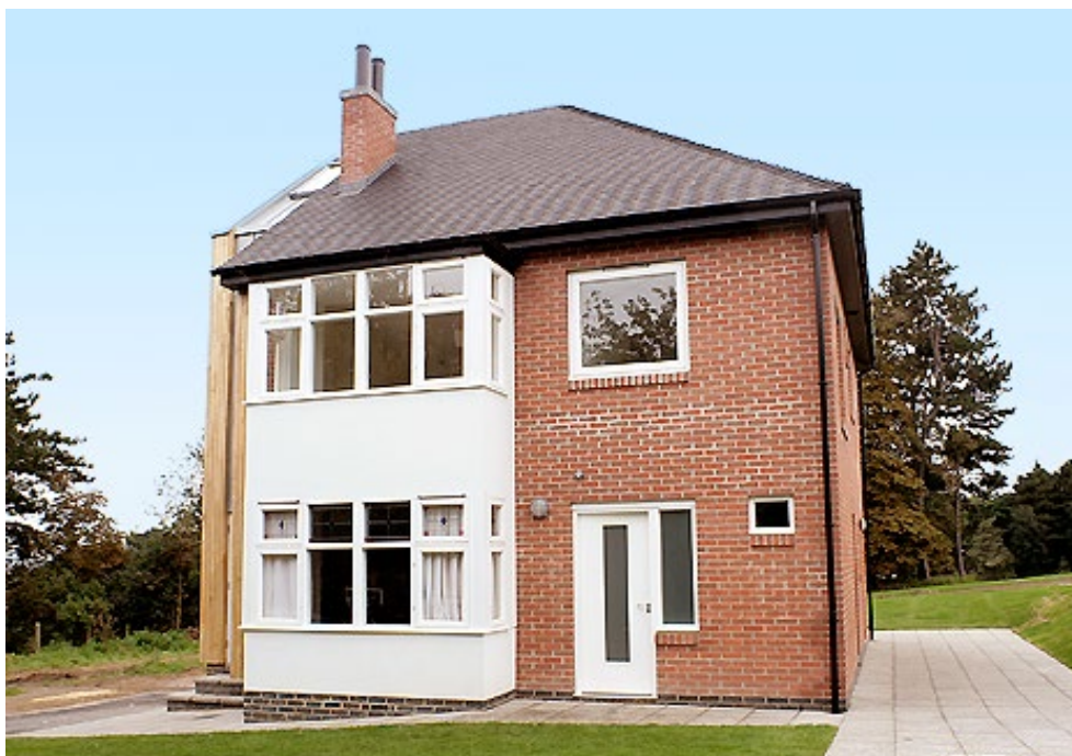
Figure 1: The CEH 1930's house with ancillary structure shown to the left.
