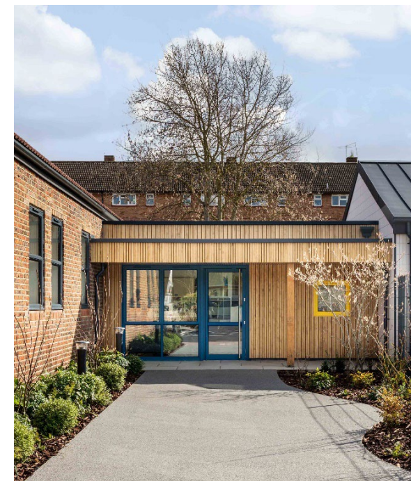
Figure 9: Level access should be provided to create a seamless and accessible route across the site for all users
