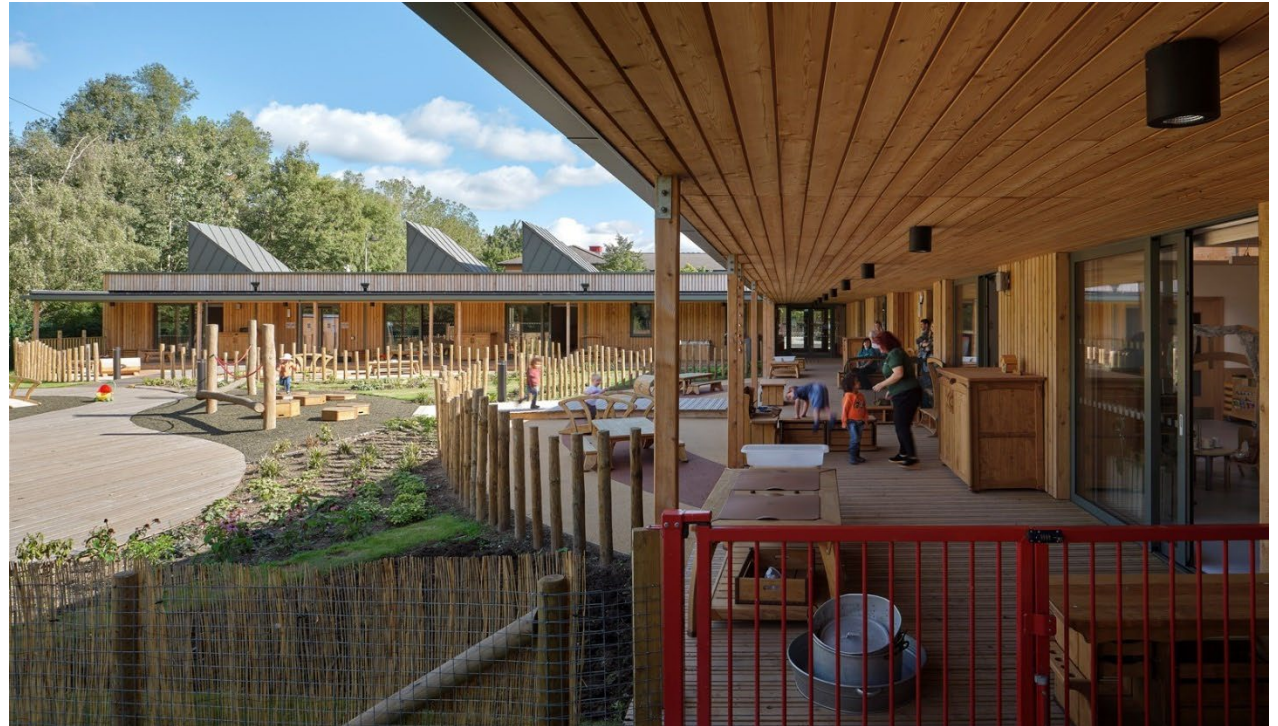
Figure 29: Immediate access from inside to outside is created with a level threshold and generous double doors. The canopy made from natural materials provides shelter from sun and rain, and houses flexible play equipment
