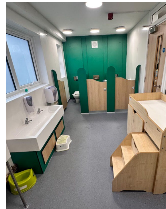
Figure 25: Washrooms should be directly accessible from playrooms and within easy reach of outdoor play. Basins and toilets sized for children to enable independent clean up
