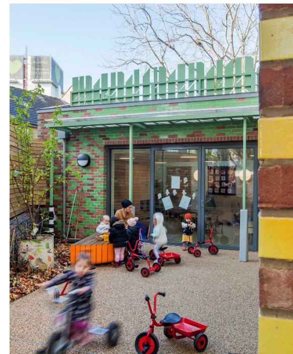
Figure 28: Free-flow between inside and outside spaces creates flexibility for children to play and supports independence
