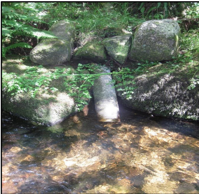
Image 7: Bywash pipe (May 2018)
