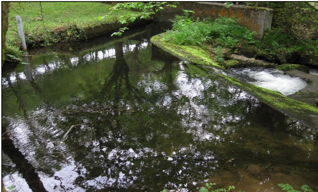
Image 3: Looking downstream to the leat, sluice gate and weir (May 2018)
