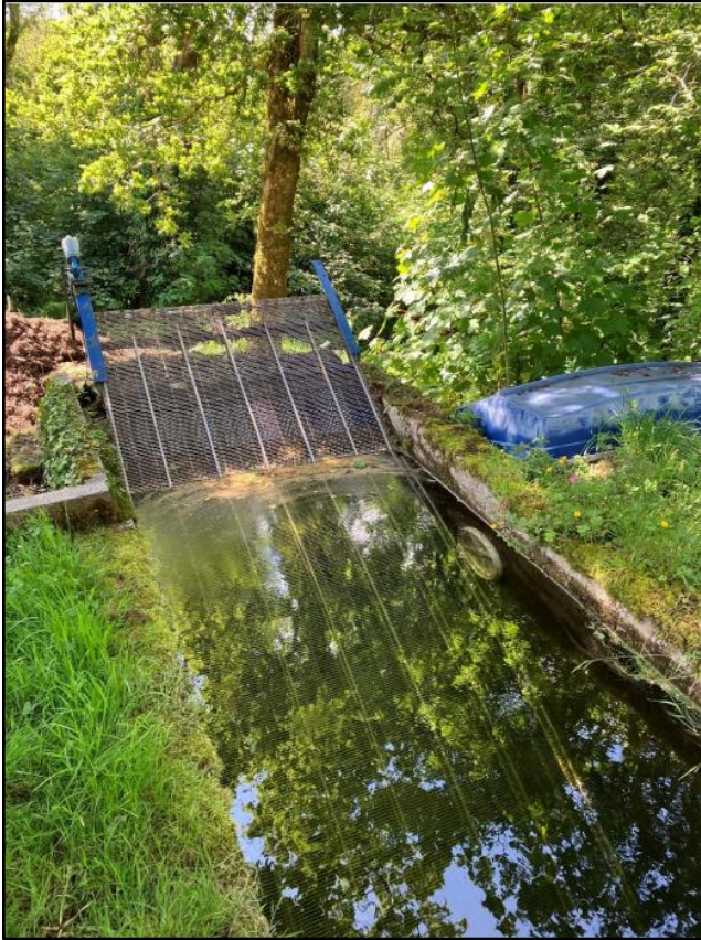
Image 4 - Existing Screen and bywash entrance (at low leat flows) June 2024
