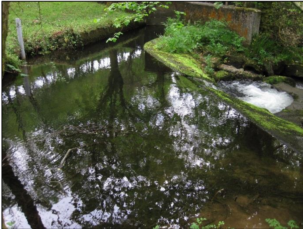
Image 1: Looking downstream to the leat, sluice gate and weir (May 2018)
