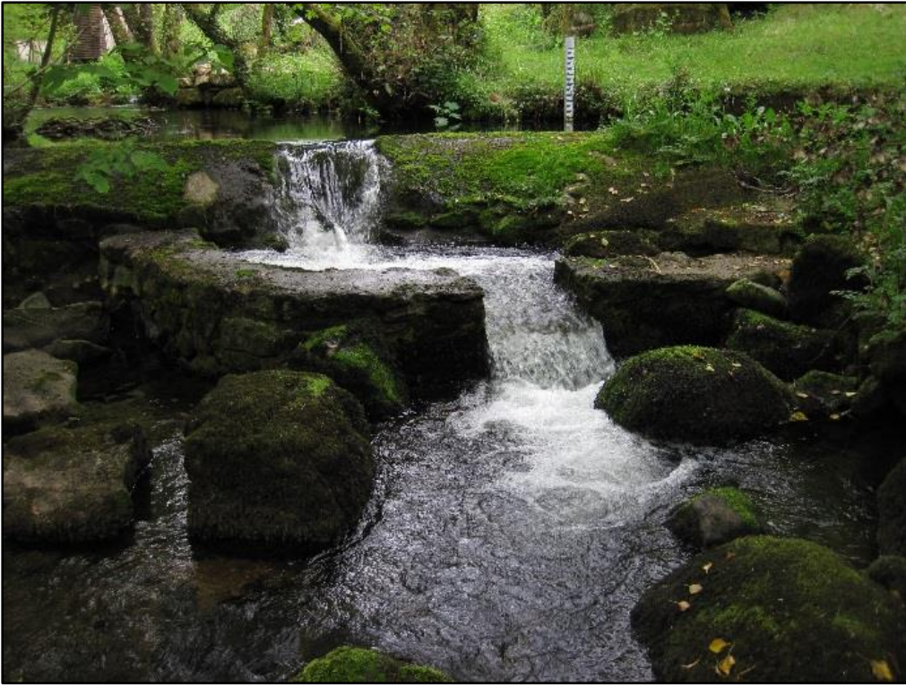
Image 2: Looking upstream to the weir on the main river (May 2018)
