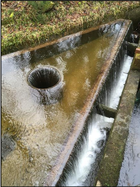
Image 5: Overflow structure shortly downstream of offtake.
