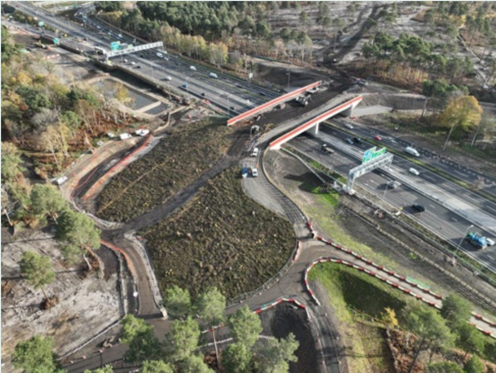
Figure 7: Cockrow Green Bridge (Source: National Highways)
