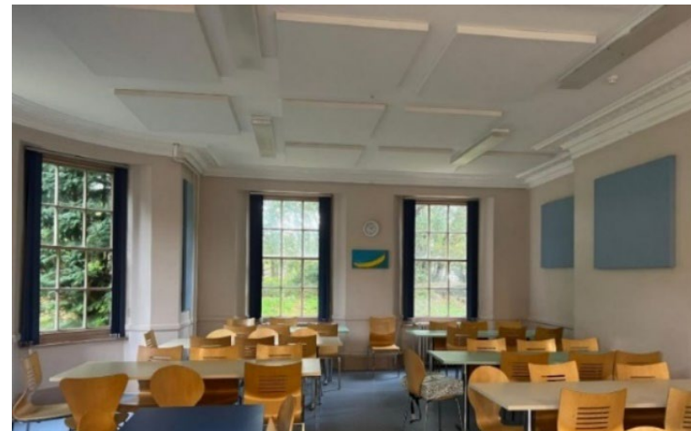
Figure 7: Acoustic wall and ceiling panels in dining space
