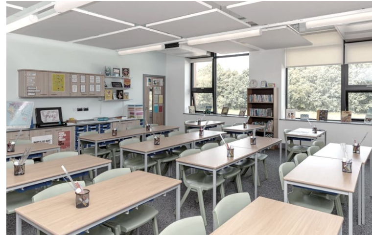
Figure 6: Acoustic ceiling panels in a primary classroom
