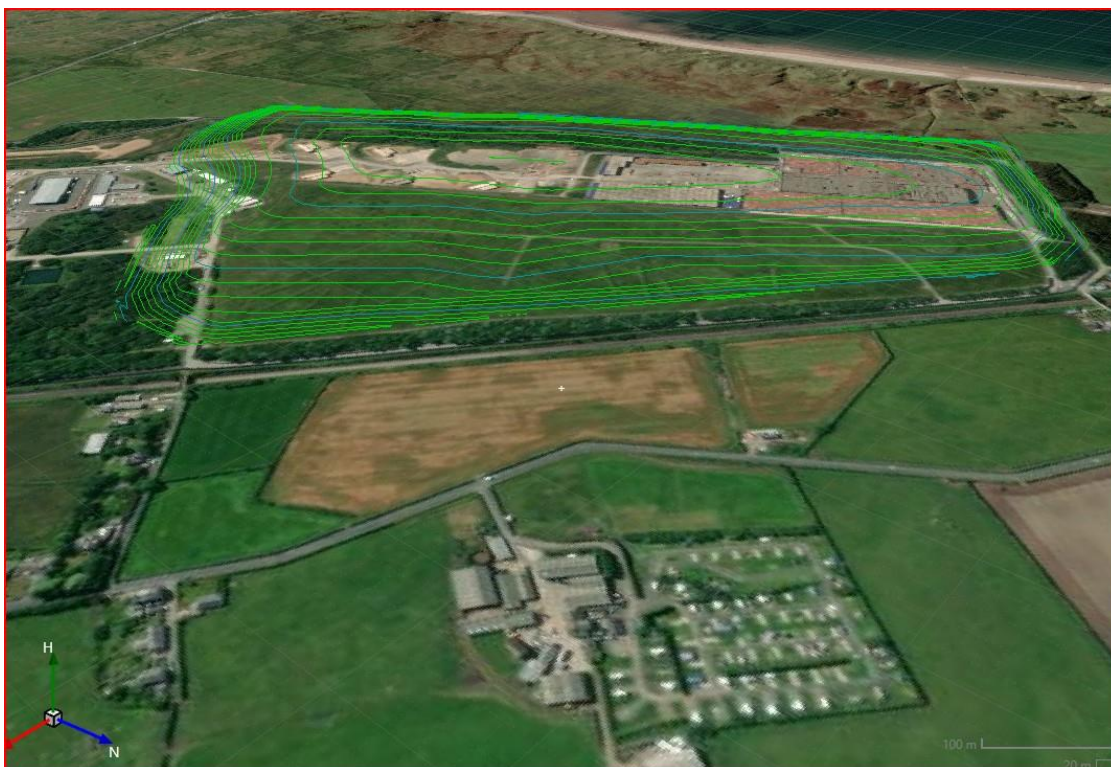
Figure 3.10: Final cap completed over the repository
