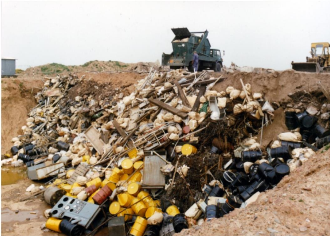
Figure 3.1: Photograph of trench disposal operations in the 1980s
