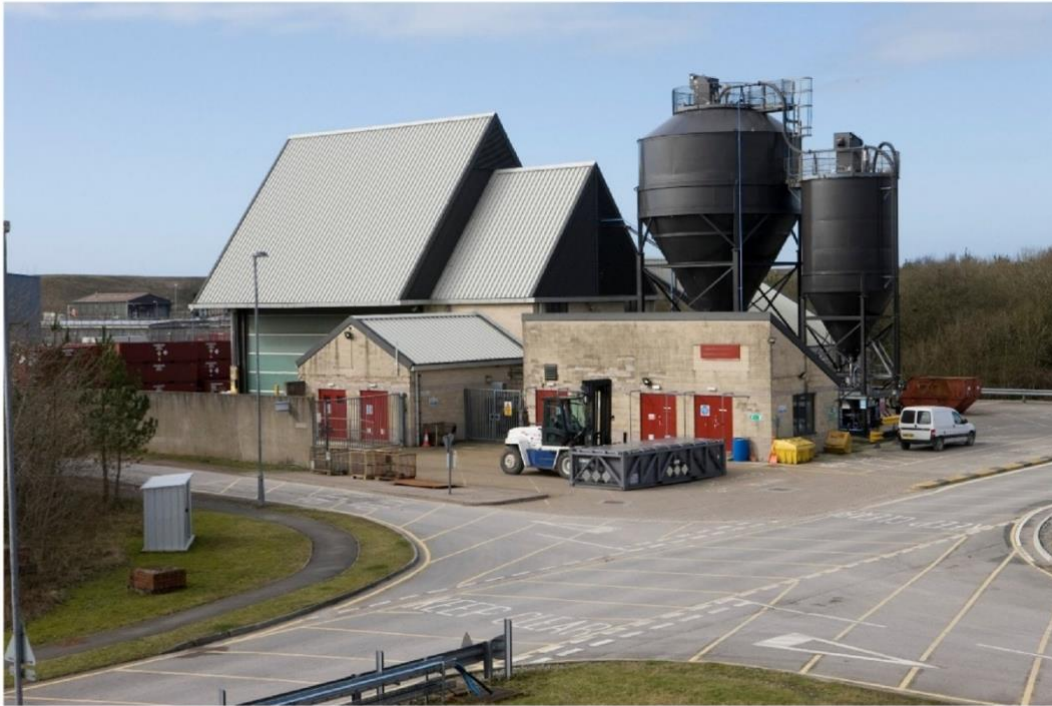
Figure 3.3: Drigg Grouting Facility
