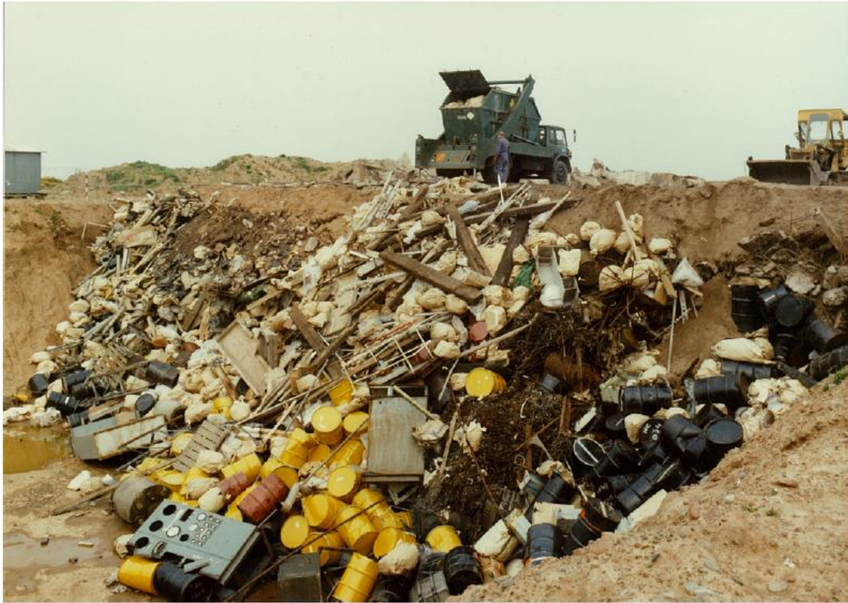
Figure 3.1: Tumble tipping of trench waste in the 1980s
