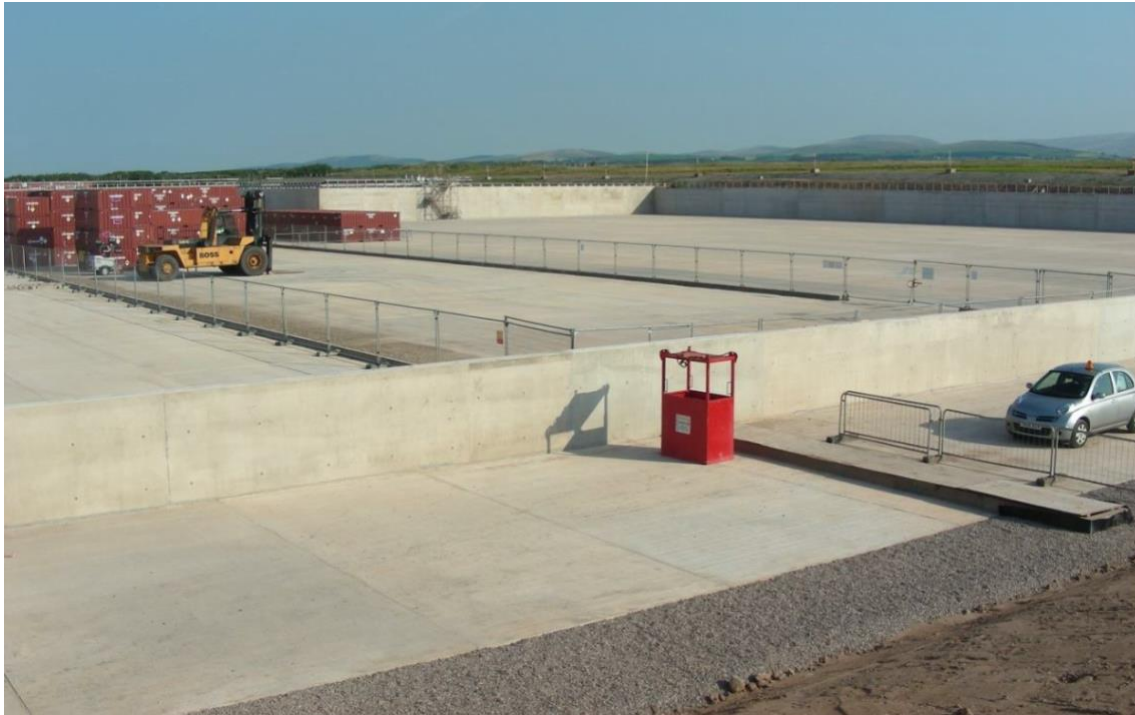
Figure 2.6: View of the base and walls of Vault 9 [22]
