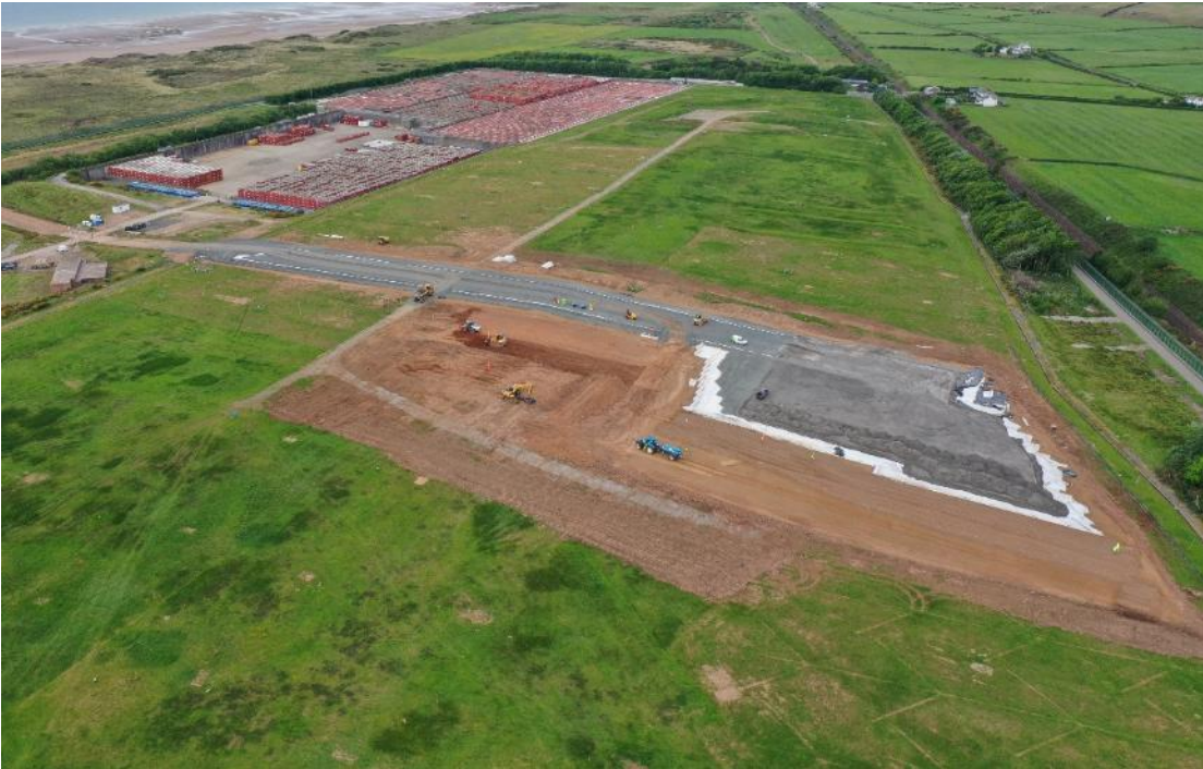
Figure 4.7: Progress on STIM including GCL Panels (site view from south)
