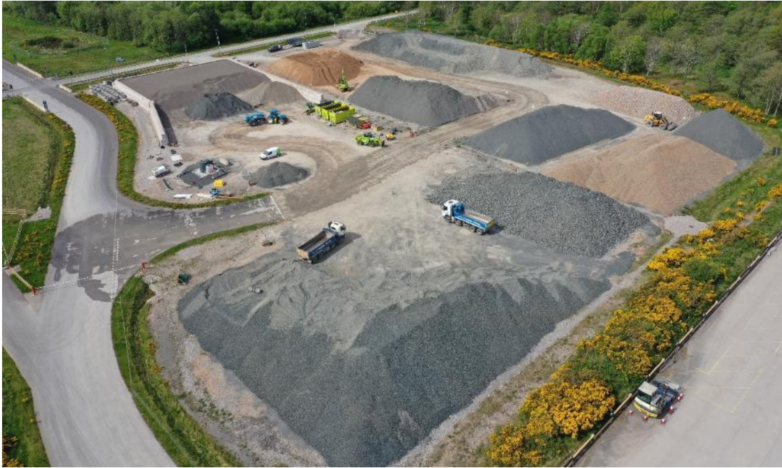
Figure 4.9: Example of Progress on STIM Supporting Works: Stockpile D
