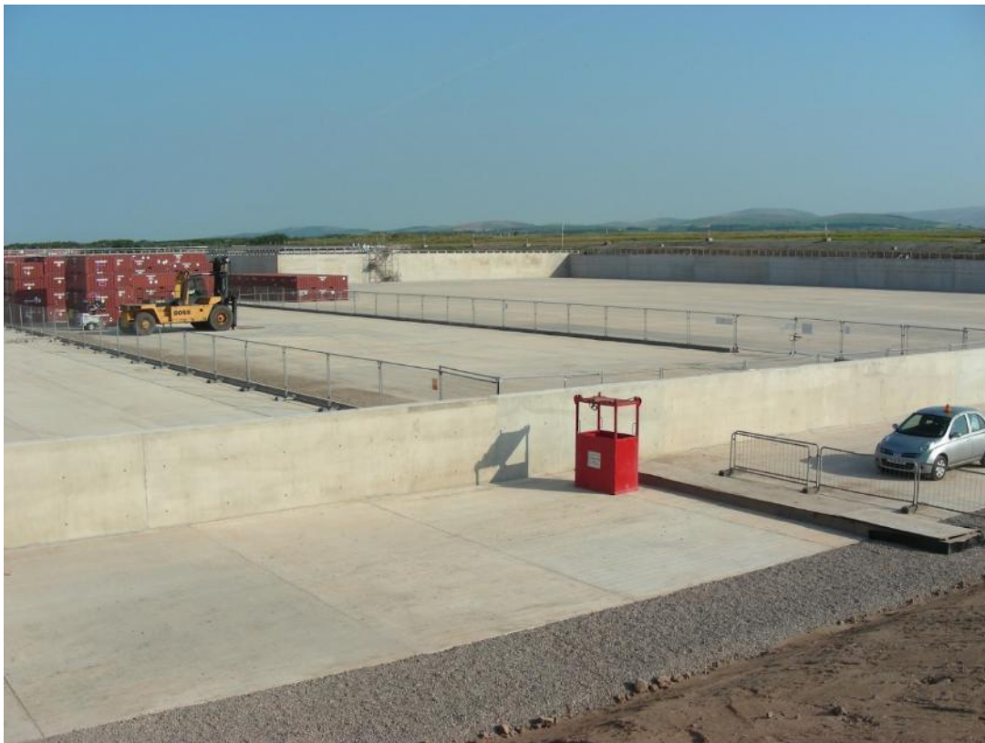
Figure 5.7: Vault 9 – view as completed
