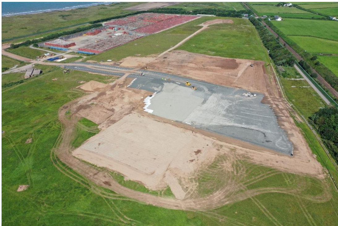
Figure 2.21: Aerial photograph from July 2025 showing work on the trench cap
