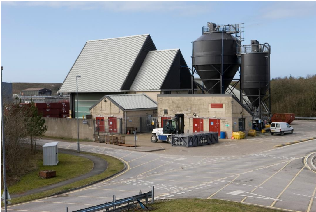
Figure 2.13: Drigg Grouting Facility
