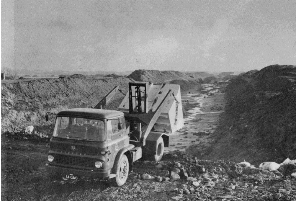
Figure 2.7: Photograph of trench disposal operations in 1961
