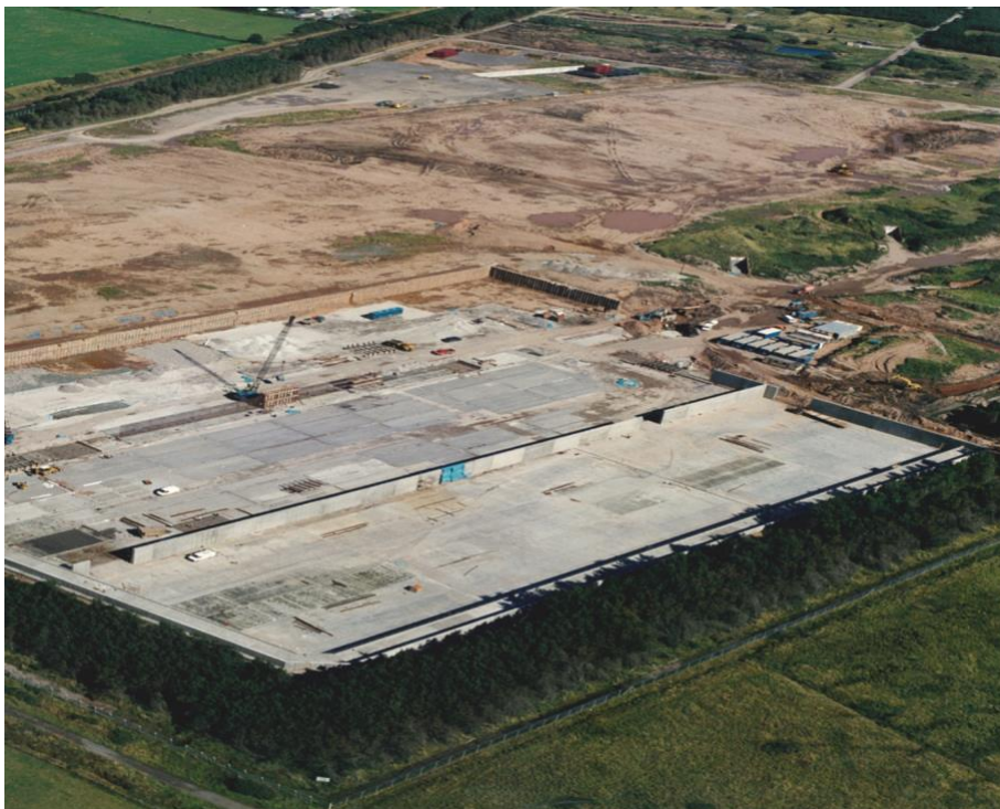
Figure 2.11: Construction of Vault 8 and capping of Trenches 1 to 6
