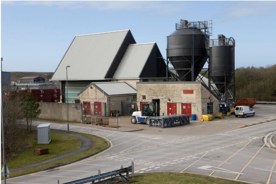
Figure 2.4: Drigg Grouting Facility
