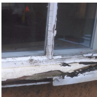
4 Condition of the wood to the windows
