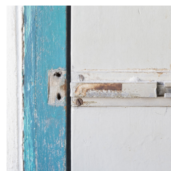
8 Broken bolt to bathroom door
