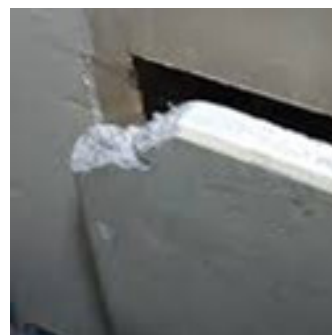
5 Damaged asbestos boxing-in
