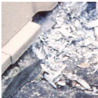
4 Close up of damaged wall panel and asbestos fibres
