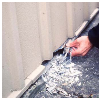
3 Damaged wall panel and asbestos fibres
