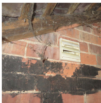
5 Extractor venting into roof void
