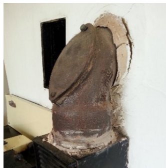
4 Cracked clay around base of flue
