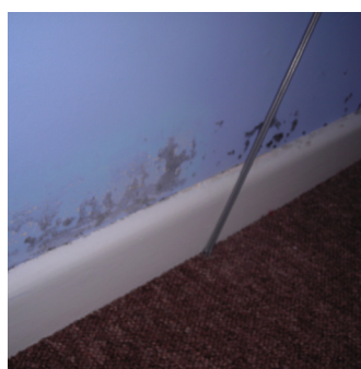
5 Mould growth in smallest bedroom
