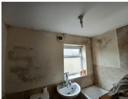
3 Mould growth to the bathroom
