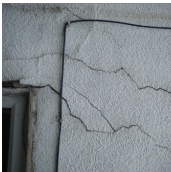
2 External wall with cracks to rendering
