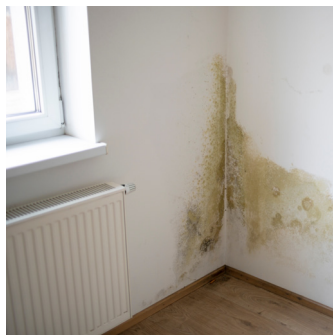
4 Mould growth to the bedroom wall
