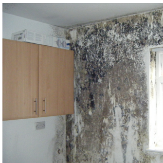
3 Mould growth to the externl kitchen wall
