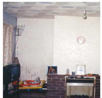
5 Mould growth to the living room wall
