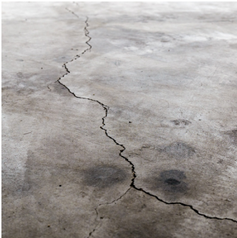
3 Crack to dining room floor
