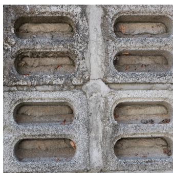
2 Blocked air bricks at the property
