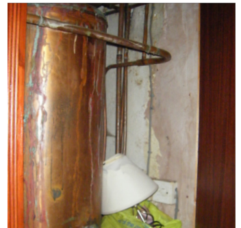
5 Uninsulated hot water tank
