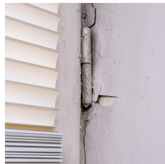
6 Damp and crumbling plaster to window reveal
