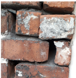
4 Damaged brickwork
