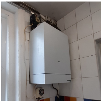
2 30-year-old non-condensing boiler
