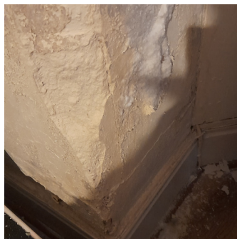
5 Damp salted internal plaster
