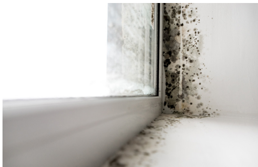
5 Mould growth to bedroom window reveal
