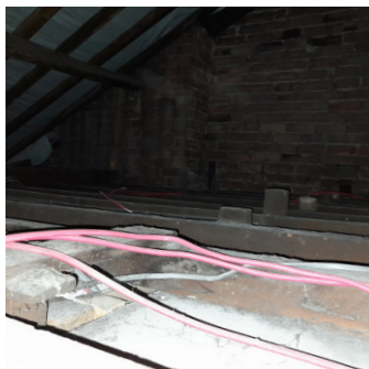
3 Loft space lacking in insulation
