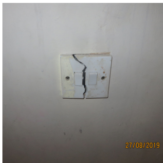
3 Cracked light switch to kitchen
