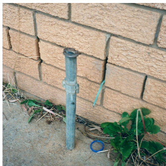
3 Earthing not attached to copper rod Photo credit: Healthabitat
