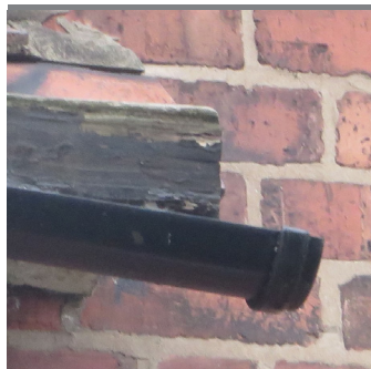
4 Loose rear eaves gutter
