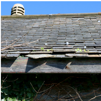
3 Roof with slipped and missing slates
