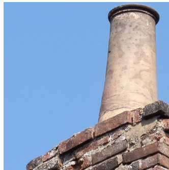
5 Disrepair to chimney
