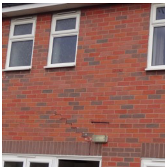
4 Crack above the kitchen window
