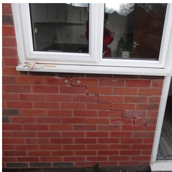
2 Crack below the kitchen window
