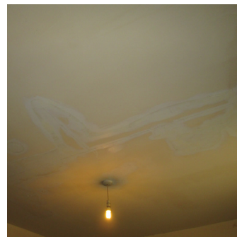
4 Water ingress and bulge to kitchen ceiling
