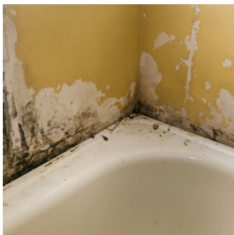
2 Failed seal around bath
