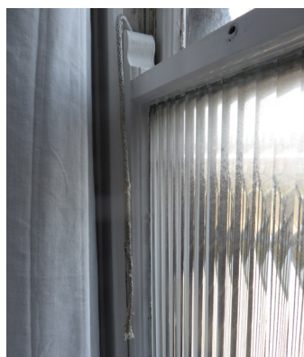
4 Snapped sash window cord
