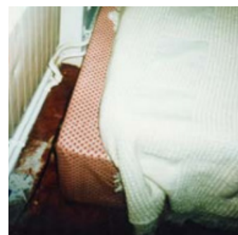
3 Gap between foot of bed and uninsulated central heating pipes
