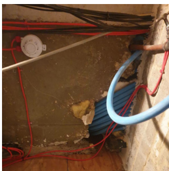
4 Penetrations to service cupboards and damaged ceiling
