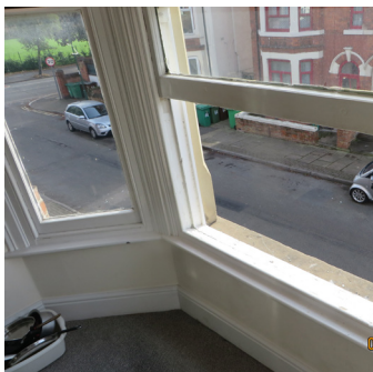
2 Sash window open with low sill height
