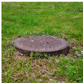
2 Raised inspection chamber in lawn
