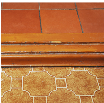
2 Raised threshold between living room and balcony
