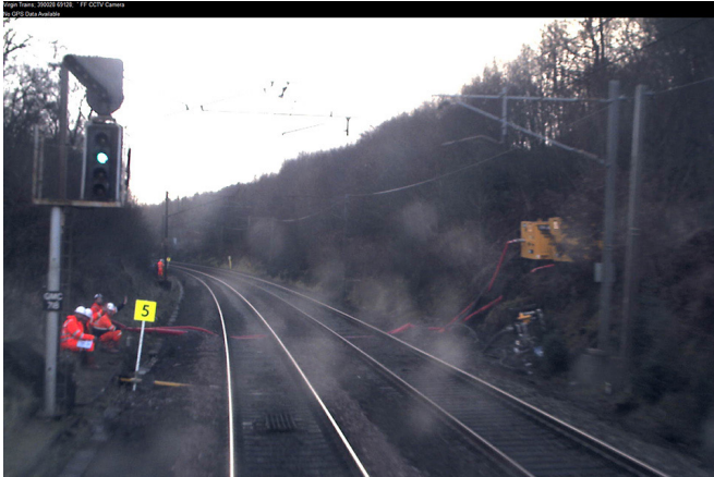
Forward-facing CCTV showing the speed indicator at the start of the ESR near Beattock.
