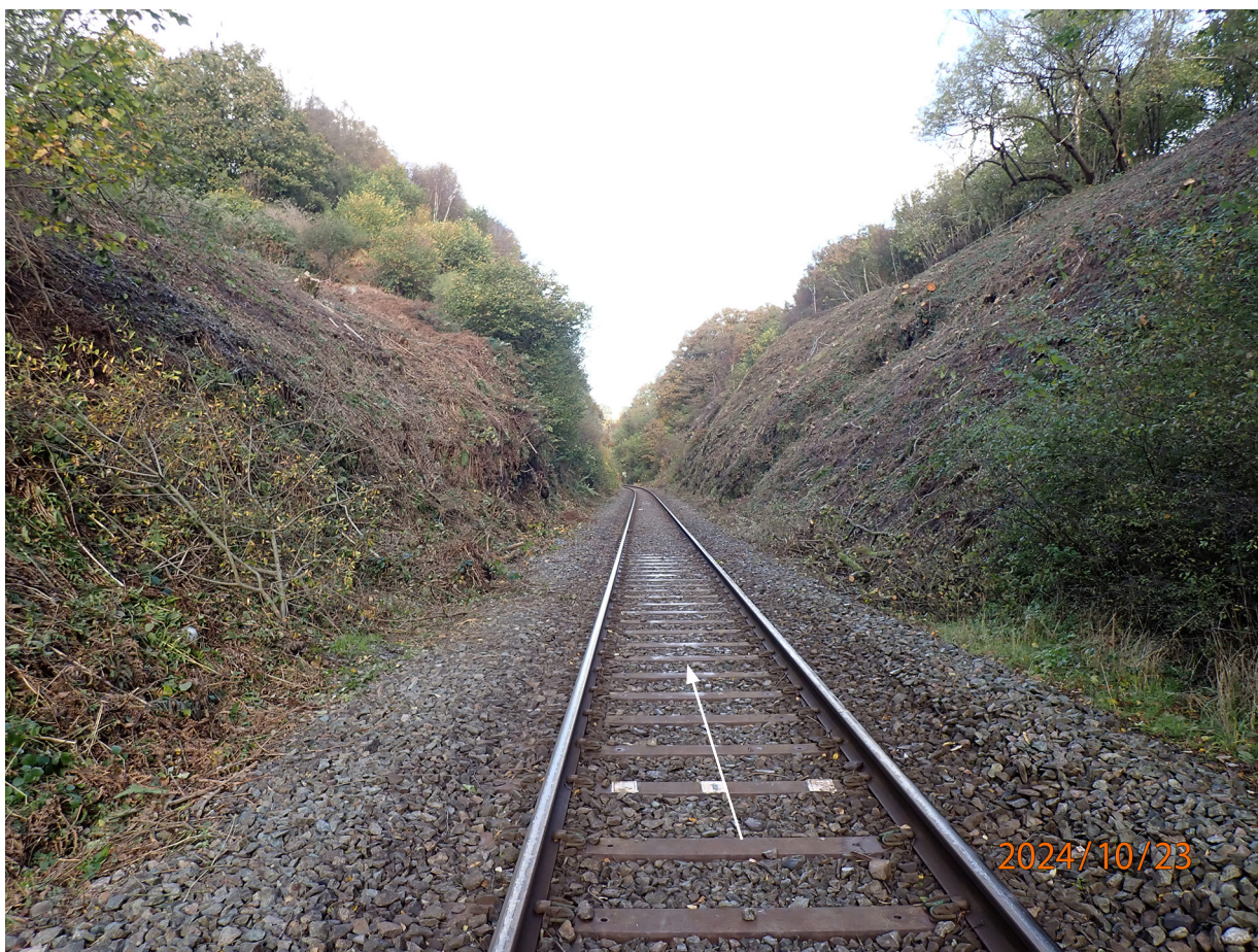
Figure 51: Lineside vegetation approximately 530 m from the collision location.
