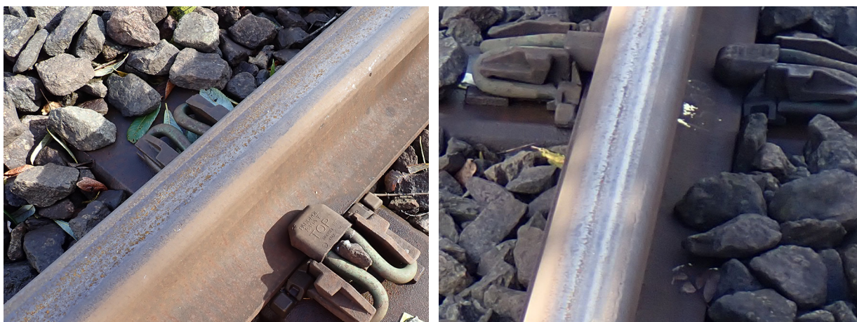
Figure 25: Example of visible contamination observed on the railhead at around 11:25 hours the morning after the accident, on the approach to the loop at 1400 metres (left) & 1500 metres (right) on approach to the point of collision.
