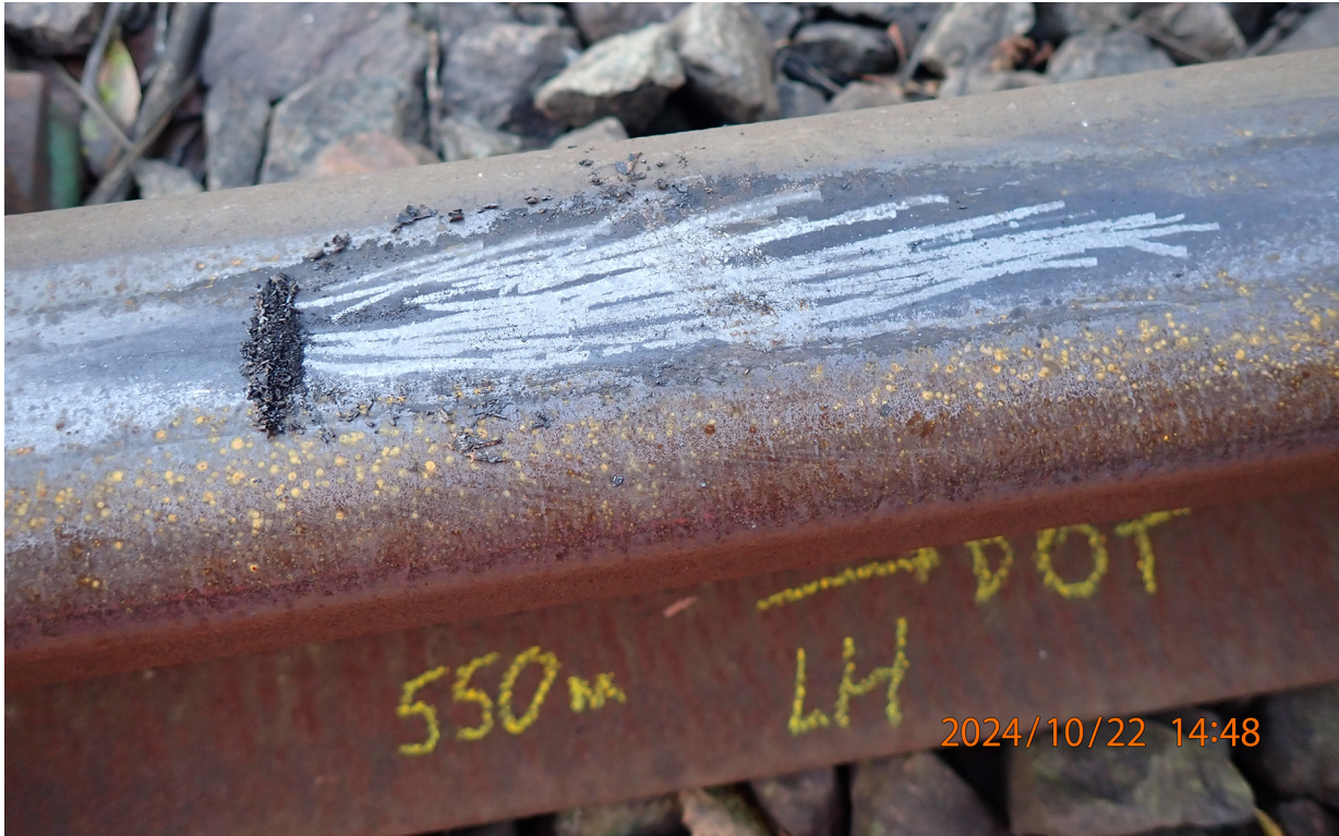
Figure 26: Example of sample collection (scraping) on the day after the accident, taken at a location 550 metres on approach to the point of collision.
