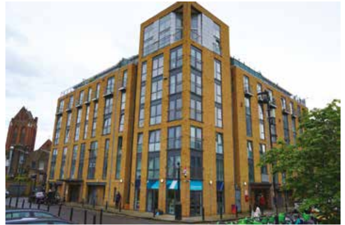
Glyn Street Estate, London - £447,546 of capital grant funding to support efficiency improvements that resulted in a 72% reduction in heat loss (photo credit: FairHeat).
