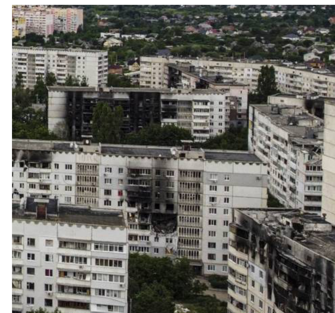
Damaged residential buildings in Kharkiv © Norman Foster Foundation
