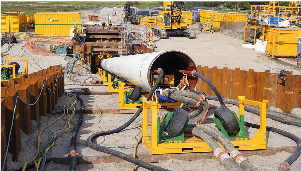
Figure 5: Direct Pipe (Herrenknecht, 2025)
