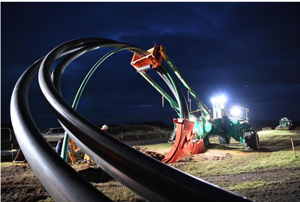
Figure 1: Cable ploughing (Thomas, 2024)
