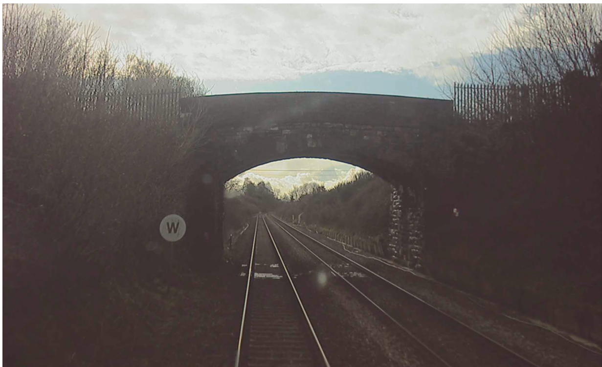
Figure 7: Forward-facing CCTV showing whistle board sign adjacent to down line near Dursden Lane bridge (courtesy of Great Western Railway).
