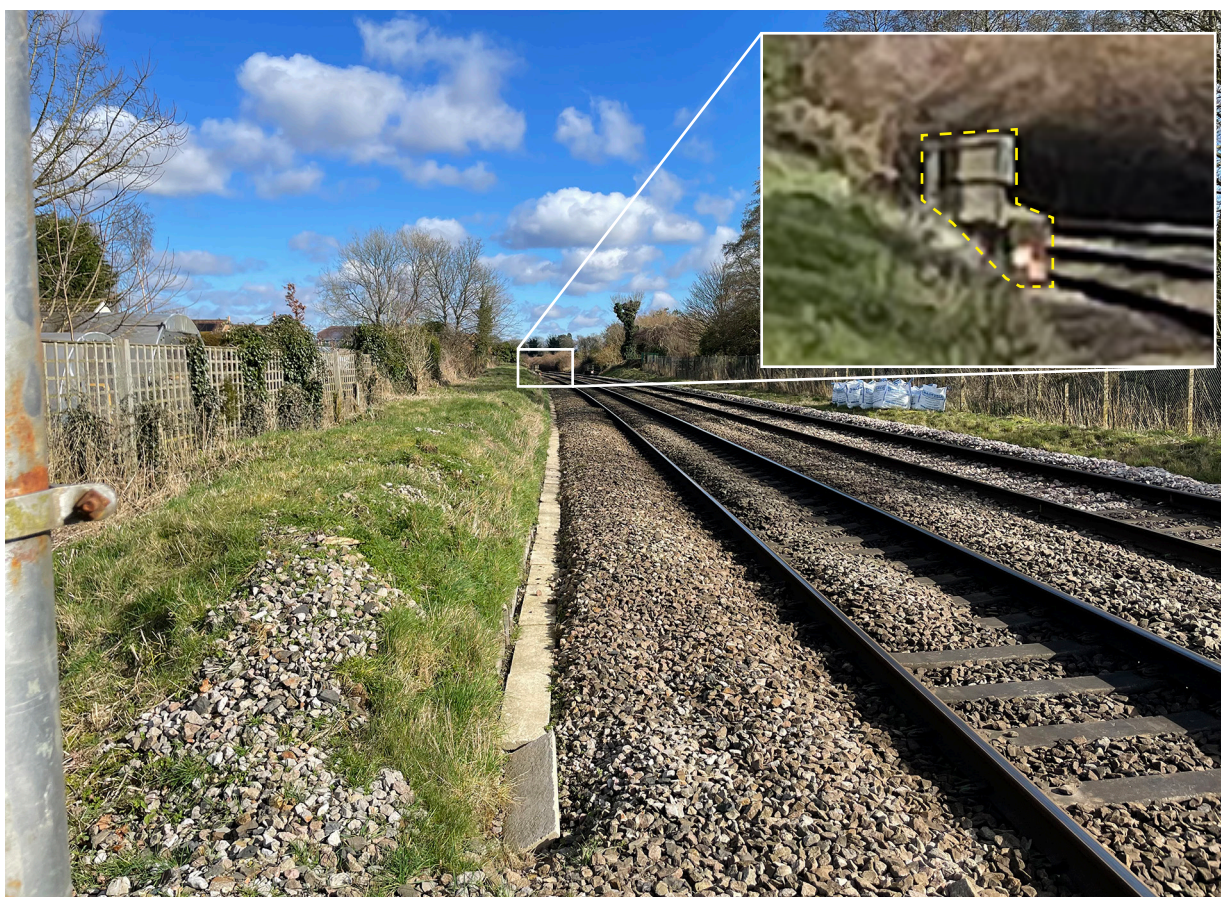
Figure 10: View from the decision point on the north side of the crossing of trains approaching on the down line. Inset image showing parapet (yellow outline) running alongside the railway, associated with the Hollybush Lane underbridge.
