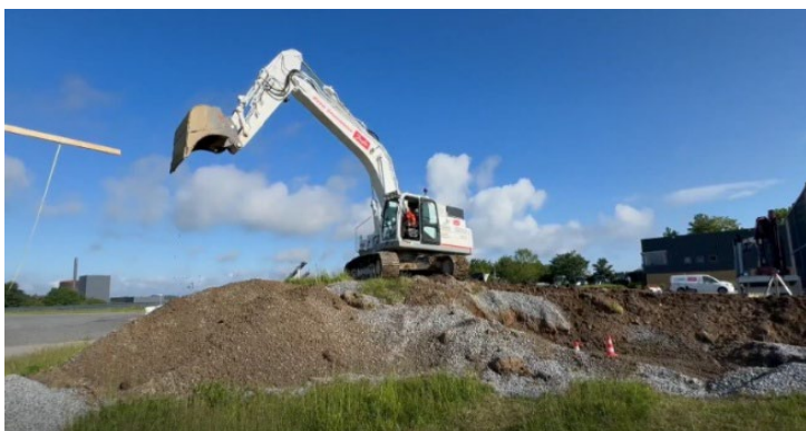
Figure 22: JCMAS air dig and dump cycle test set-up.
