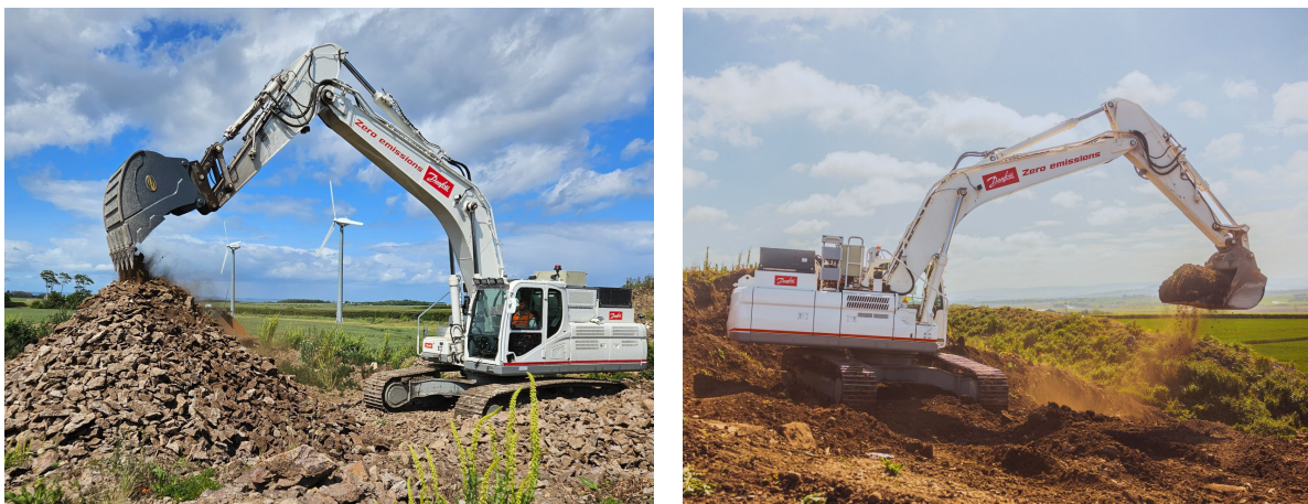
Figure 39: DEPOWER2 excavator working at FRM East Fenton
