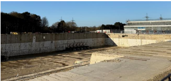
Image 2 & 3: Completed Turbine Hall Demolition
