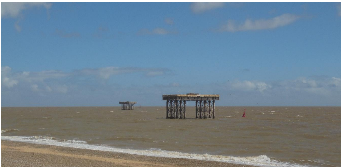
Image 7: Cooling water intake and outfall structures
