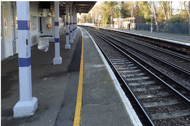
Platform with no tactile surface markings at Eden Park.
