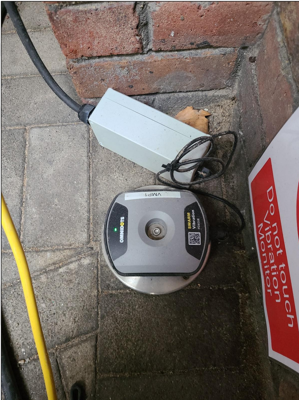
Image 2 – VMP1 Monitoring Location
